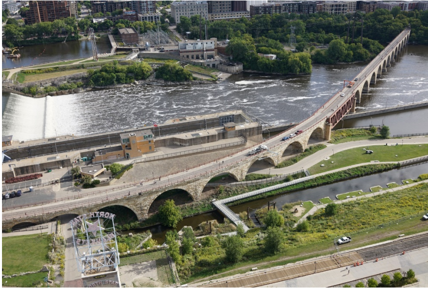
Caption: The Stone Arch Bridge Rehabilitation Project utilized unmanned aircraft system (UAS) inspection, digital twins and mixed reality. Image courtesy of Collins Engineers
