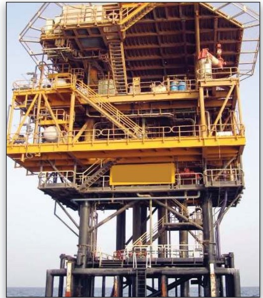
SACS simulations allowed the company to substantiate the insurance claim resulting from the accident, saving the operator considerable costs.
