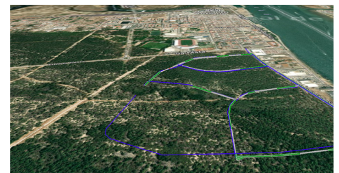
Enabling 4D digital rehearsals and real-time field data management for a coordinated sewer network construction.
