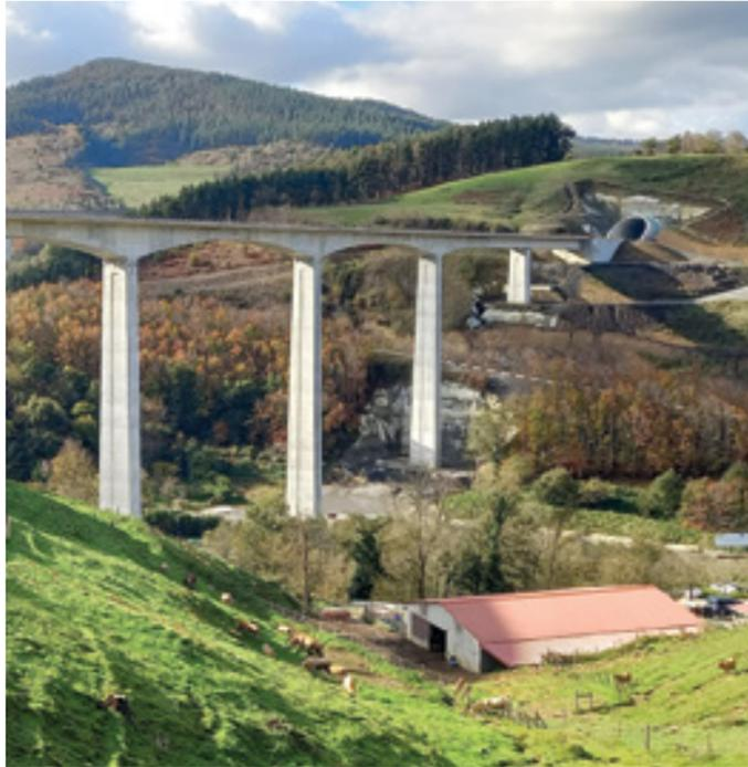
The Zumelegui viaduct is part of a new high-speed railway in Vizcaya to reduce traffic between the provincial capitals of the Basque Country and connect Spain's cities through fast, clean, and safe transportation. Spanning 481 meters in length and divided into seven spans, the deck is connected to four central piers using the balanced cantilever construction method. The project presented site and structural challenges requiring comprehensive and flexible bridge modeling and analysis technology.
