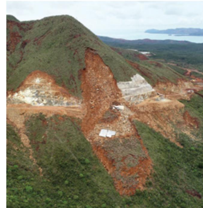
When construction of a 2.2-kilometer critical access road in New Caledonia was halted due to a landslide, engineering and construction manager Hatch initiated a comprehensive stability assessment of the area, designing a remediation plan and validating continued construction along the planned alignment. Faced with technical, coordination, and site challenges, Hatch needed a collaborative digital geotechnical solution to avoid a costly and environmentally damaging alternative realignment.
