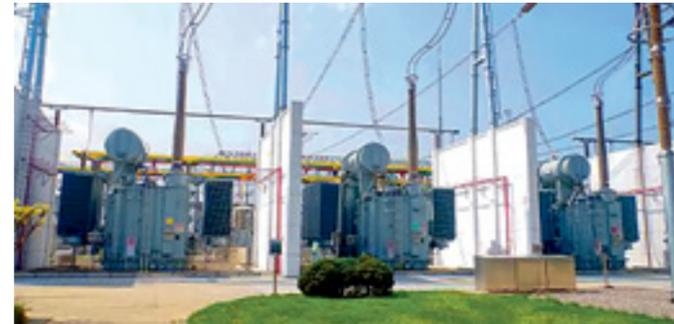
This substation expansion project featured substation frames, concrete houses, firewalls, and foundation design. With strict cost controls, a tight schedule, and full American Standard design requirements, the project presented challenges requiring digital workflows and comprehensive structural design software.
