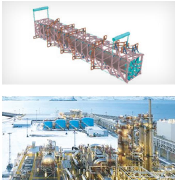
This refining and chemical integration project has an oil refining capacity of 16 million tons per year and produces paraxylene and ethylene cracking, as well as hydrogen and methane. The plant includes a refrigeration box and internal equipment that together weigh a total of about 640 tons. To consider the structural integrity during operating, lifting, and transportation conditions, the project team needed comprehensive structural design and analysis technology.
