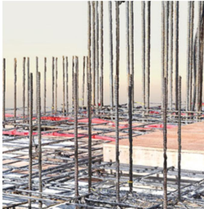
To monitor and manage on-site works and ensure correct installation of rebar for this construction project, PrimeTech implemented 3D modeling. They wanted to create a reality mesh of the site to enable remote supervision and avoid safety hazards at the construction site. The complexity of the building construction site made it difficult to use laser scanning. The team needed a flexible and robust reality capture solution.
