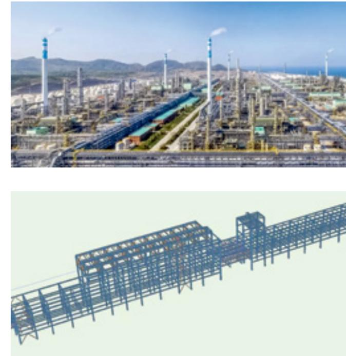
This project involved the structural analysis of the main pipe bridge of a refinery in South China. The structure is 220 meters long and six stories tall, with its highest point reaching 21.5 meters. It is equipped with two spanning trusses and localized air coolers. Bearing heavy loads, the structure required assessment to determine its structural integrity. The team realized they needed comprehensive structural analysis and design technology to successfully deliver the project.
