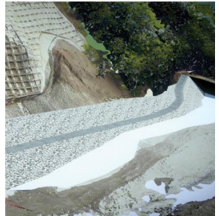
Located at an altitude of 1,200 meters in the upper reaches of the Komu River is a mountain road leading to the three peaks of Mount Hoo in Yamanashi. To help prevent erosion and landslides, the R2 Komu River Upstream Bank Protection project was initiated, requiring significant earthworks and temporary construction. The narrow, winding road sees many animals that can jump out suddenly and potentially cause falling rocks, presenting dangerous on-site working conditions.
